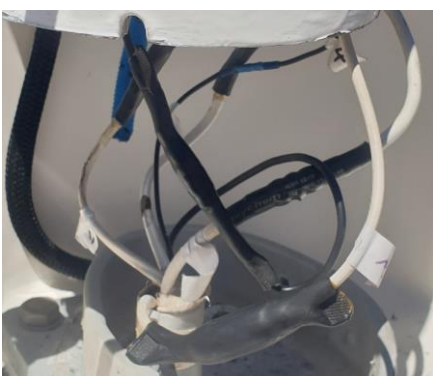
New wiring at mast base
